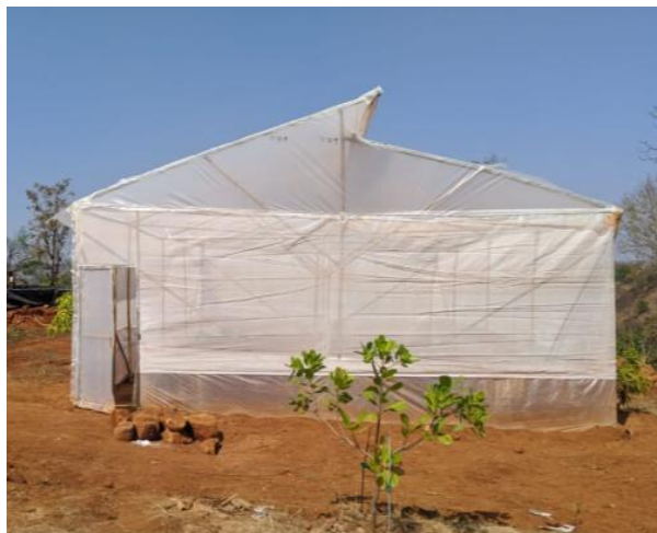
Fig. 4 (a): Bamboo polyhouse installed at Ramkhind village (Polyhouse 1)
